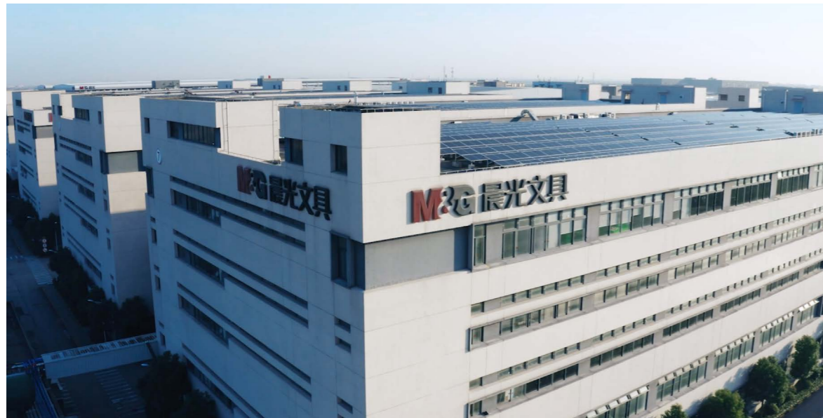
Rooftop photovoltaic power generation units at M&G Shanghai base
